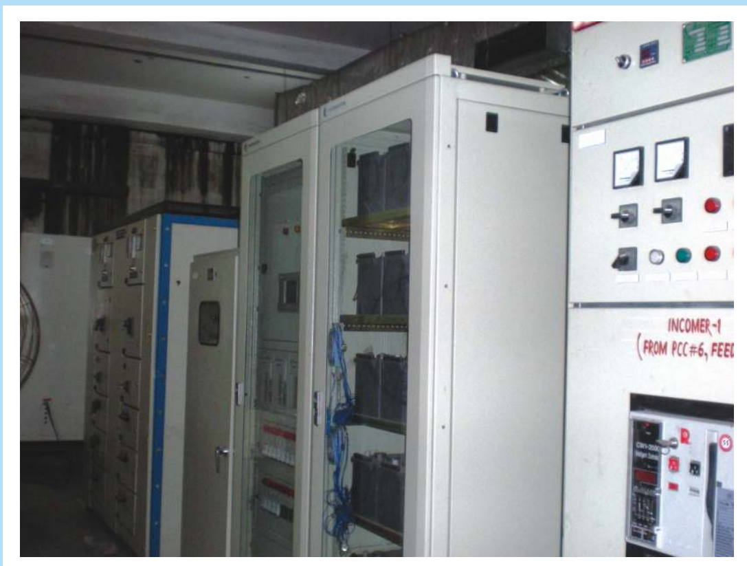
Central Electrical Work at JSPL Raigarh Contract No.4778001057
