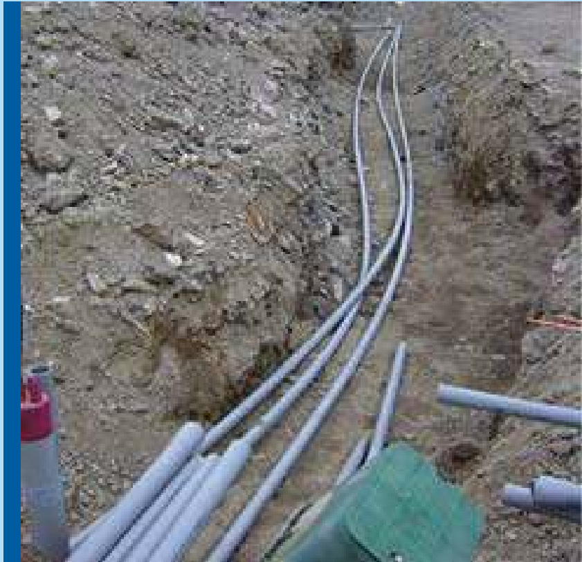
Cable Laying work at PP3 Electrical at JSPL Raigarh Contract No.4978000325
